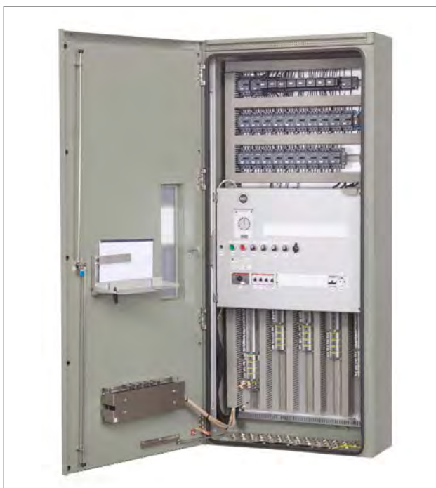
Figure 16. ETOS® control cabinet
